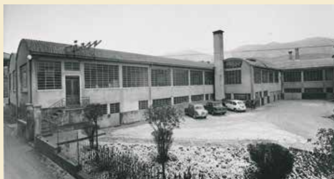
Primera fábrica de Cimberio, 1957 Cimberio's first manufacturing facility in 1957
